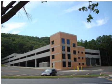
The existing parking deck accommodates 390 cars.
